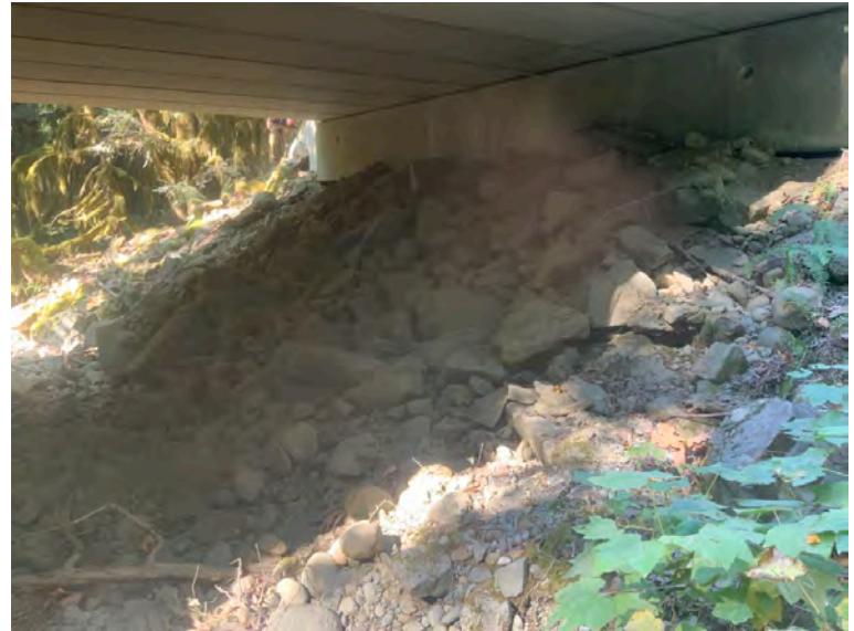
Right Bank Abutment when facing downstream
