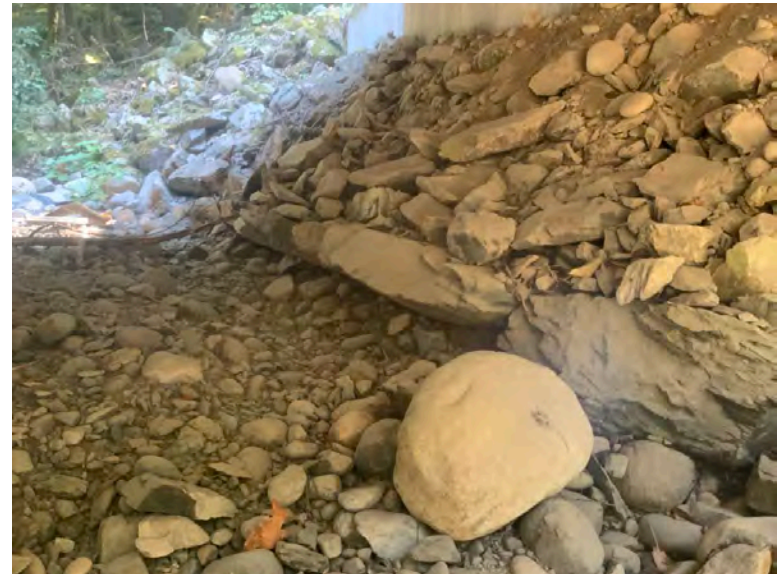
Left Bank Abutment when facing downstream
