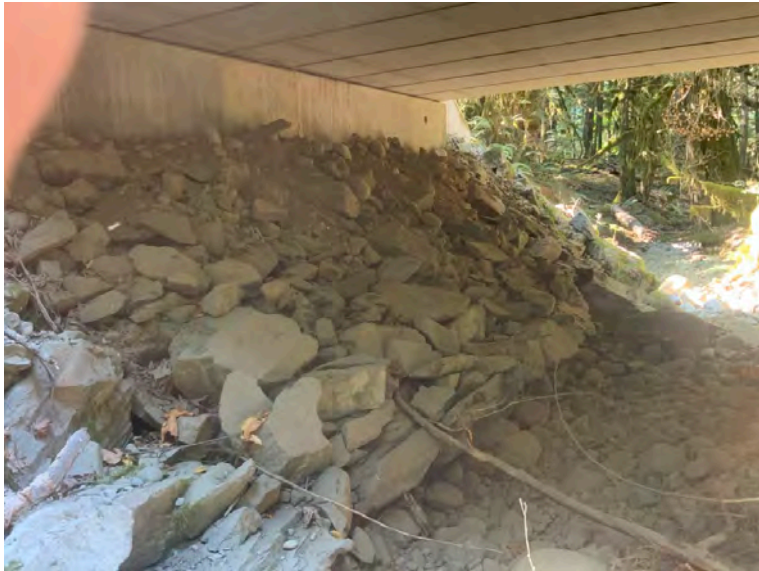
Left Bank Abutment when facing downstream
